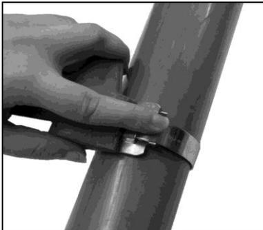
4. Place finger on BAND-IT Band at buckle bridge while tensioning. When you observe the band stops moving through the buckle, *maximum pressure is being exerted* around the workpiece. *Stop turning handle.*
